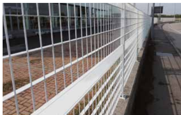
Special profile "C" section sized 80x40x23x12x2 mm
