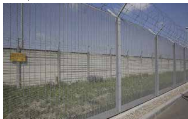
Omega post 60x40x25x3 mm 120x60x30x3 mm with cover plate
